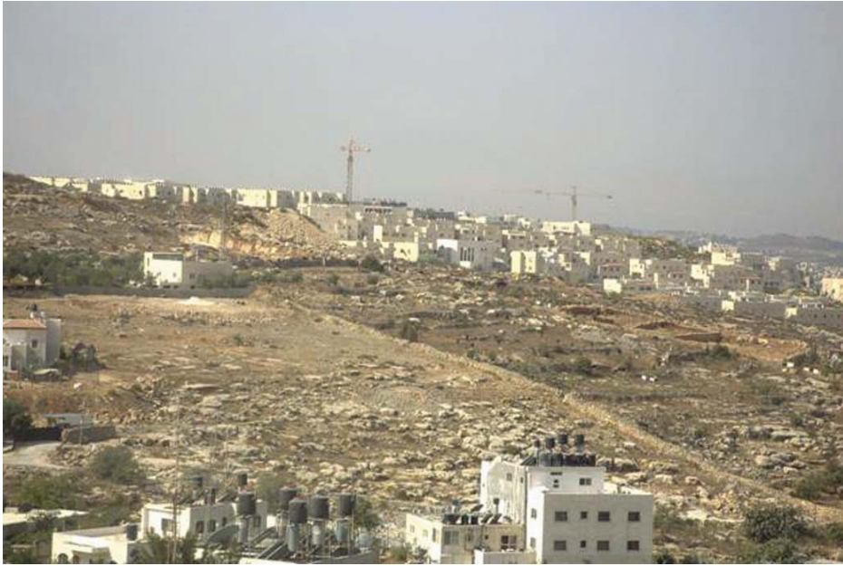
Figure 13: Shows an “illegal” house looking towards a “legal” settlement built on the confiscated land of its owner.
